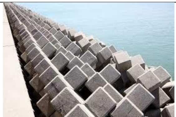
Figure 2 Breakwater with concrete shaped blocks
