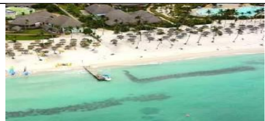
Figure 5 Picture of submerged breakwaters
