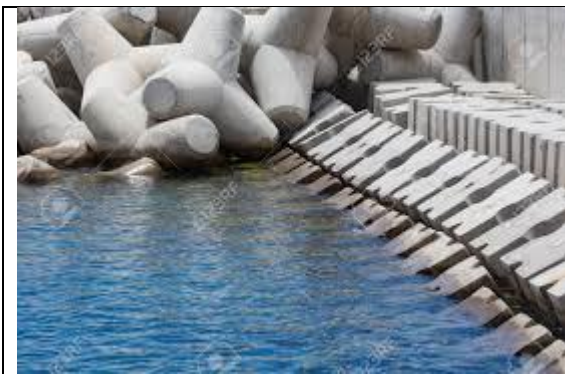
Figure 1 Breakwater with concrete shaped blocks
